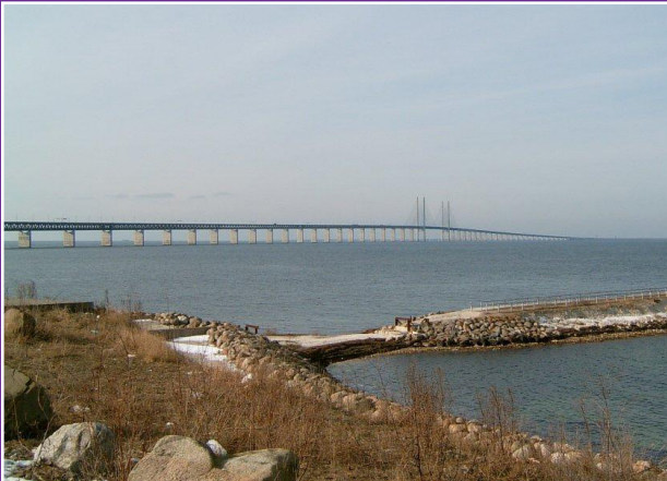
The Öresund bridge, Malmö–Copenhagen
